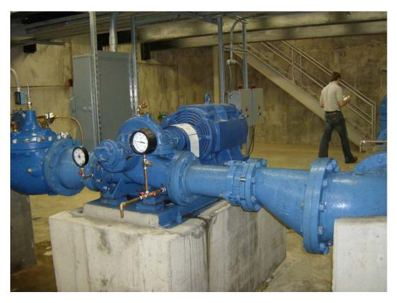
As the right edge of the picture shows, the pump's suction piping had a horizontal elbow immediately before the pump.
