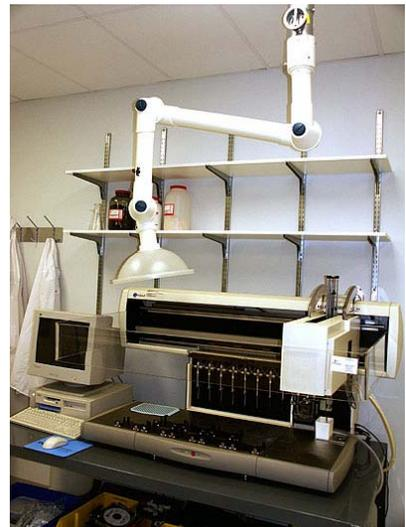
A ceiling-mounted extractor arm is readily accessible in a laboratory.
