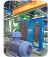
This plate heat exchanger will be used for process cooling in a power plant. Plate-and-frame heat exchangers will perform well while requiring less floor space and maintenance in many process applications.
